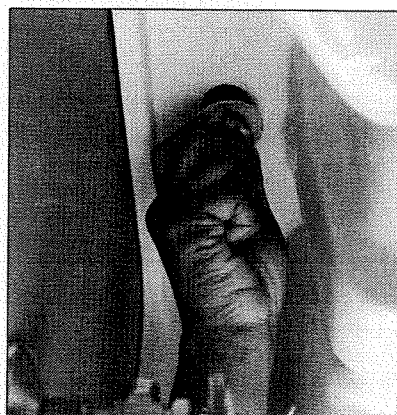
Channel for pop-up drain lever
